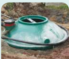
IPC access lid during installation
